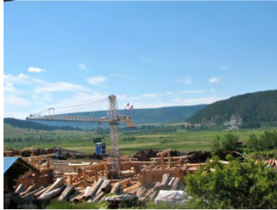
Log cabin factory
