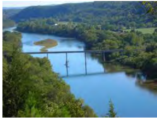
Looking at the bridge we're about to cross
